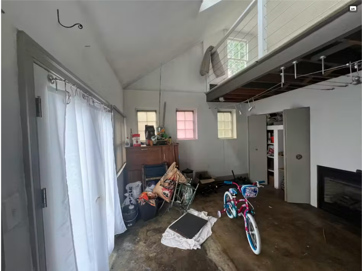
Before the renovation, the garage served as extra storage for the homeowners.
